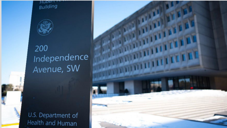
The Hubert Humphrey Building, headquarters for the U.S. Department of Health and Human Services (HHS)
